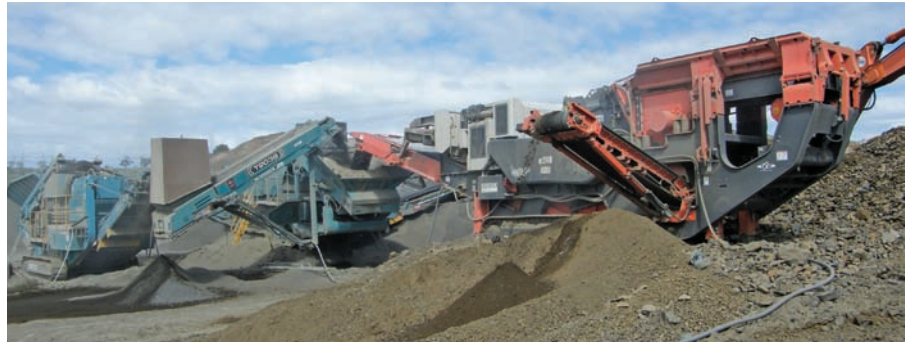
With a cleaner operation, the contractor has been able to deliver a higher spec concrete aggregate for Hi-Quality Group.
